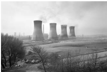
John Davies, Agecroft Power Station, 2006
